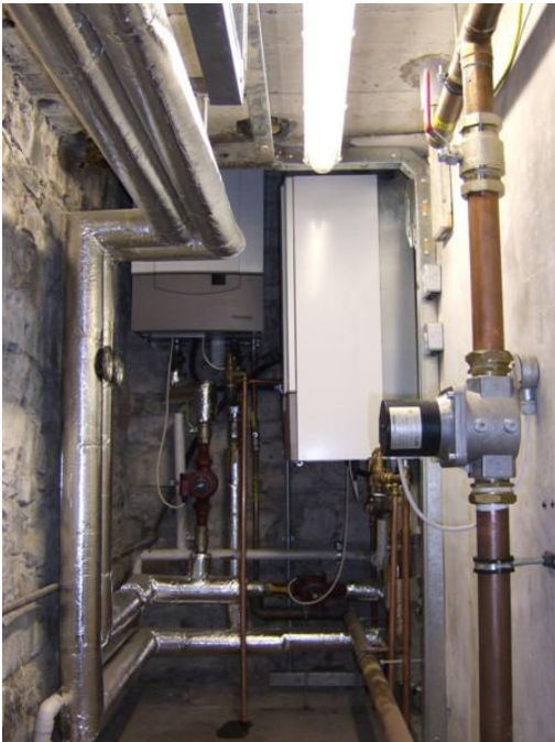
Left: The two boilers (far end of picture) Right: The pipework, pumps and valves under the Church
